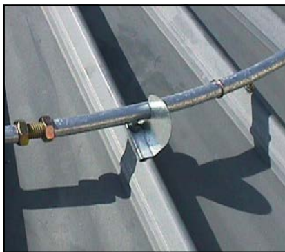
Roof Compression Rings provide additional structural support and another level of safety for those working on top of the bin.
